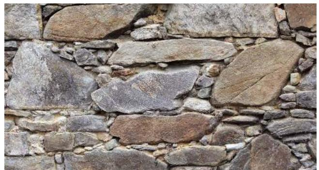
Stacked stones with pinnings deliver gravity forces to the ground.
