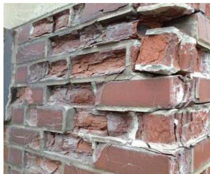
An example of spalled brick yet intact mortar.
