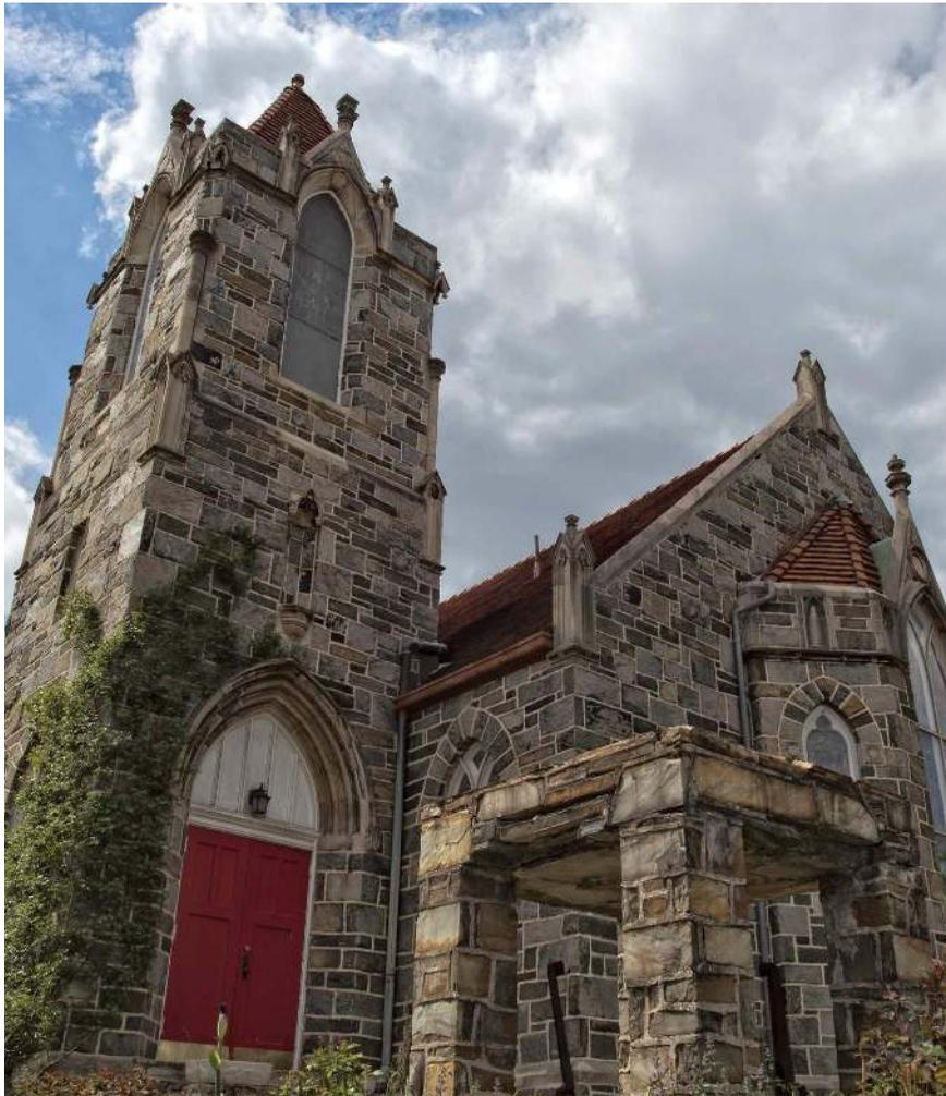
While the initial cost is high, repointing of historic masonry walls should not be postponed in favor of less expensive applications of vapor-blocking repellants, which can cause deterioration by trapping moisture.
